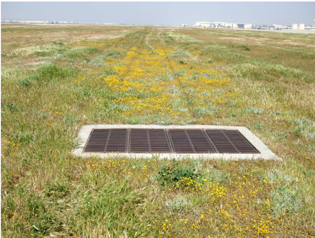
Photos 13 (above) and 14 (below) (April 2009): Shallow drainage swale adjacent to runway in Survey Area 3. Runoff from the pavement goes into the drainage swale (Photo 13) and is directed into storm drains within the swale (Photo 14). The swales are dominated by upland grasses and forbs and are periodically mowed.
