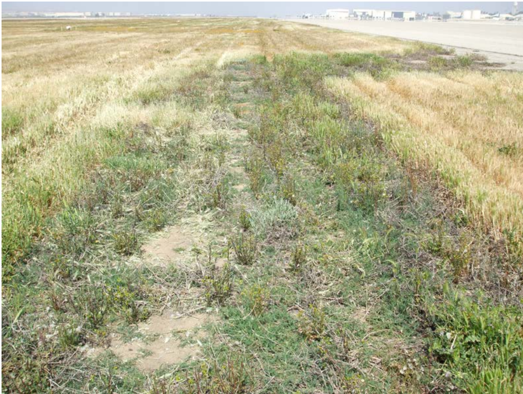
Photos 13 (above) and 14 (below) (April 2009): Shallow drainage swale adjacent to runway in Survey Area 3. Runoff from the pavement goes into the drainage swale (Photo 13) and is directed into storm drains within the swale (Photo 14). The swales are dominated by upland grasses and forbs and are periodically mowed.
