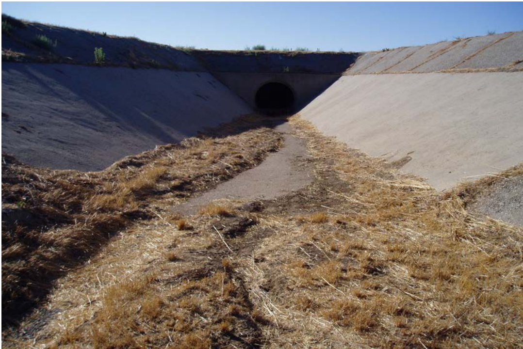
Photo 5 (October 2006): Concrete lined channel in the main drainage in Survey Area 13. Debris and sediment collected at the base of the channel and patches of wetland plants had established on top of the sediment. Water flows into an underground culvert at the end of this channel (slightly visible in the shadow).
