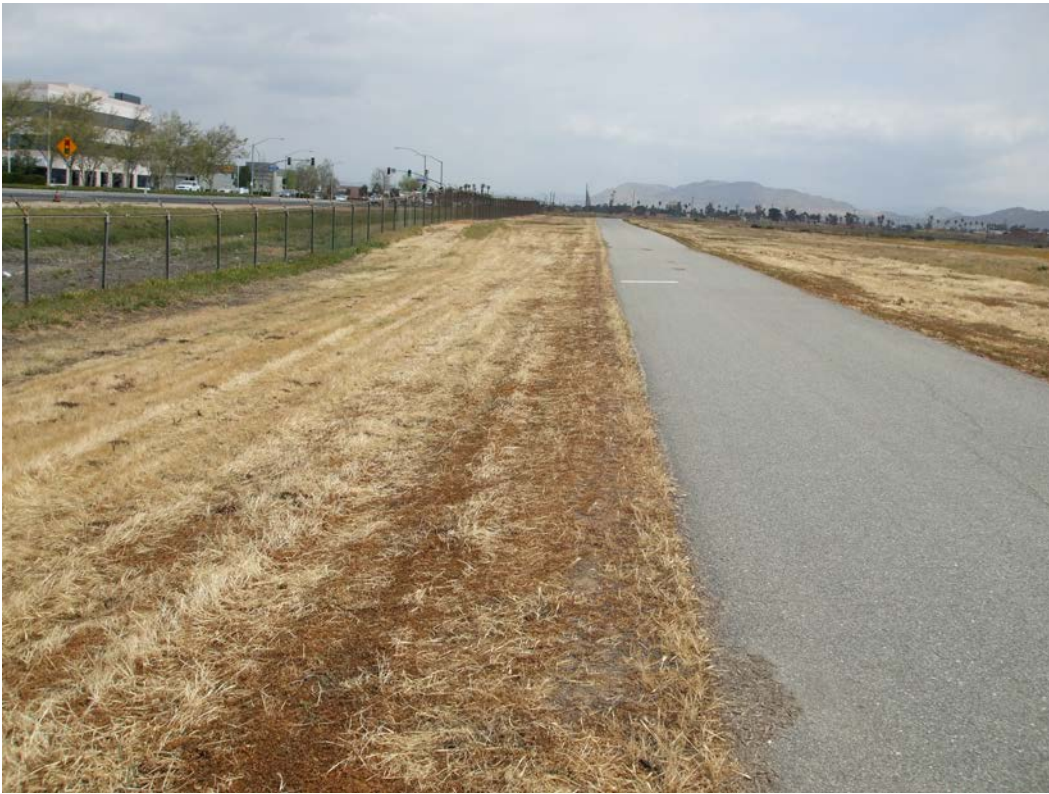
Photo 9 (April 2009): The Cactus Avenue Flood Control Channel is outside the March ARB northern boundary fence, but a portion of the channel in Survey Area 5B is fairly flat and wetland vegetation (green band of plants along the fence line in the photo) and saturated soils extend into Survey Area 5A.
