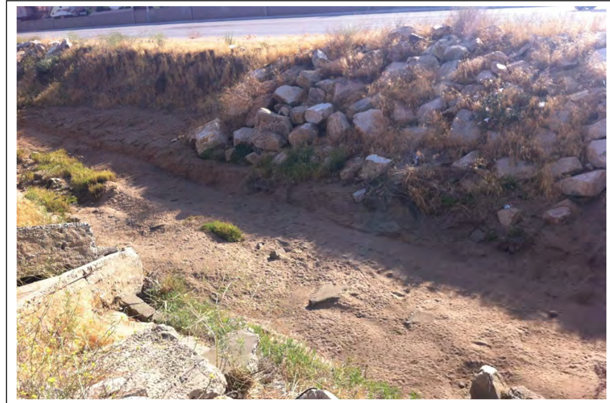
Photograph 4: View looking northeast, just north of Meyer Drive. The photo represents area of unvegetated streambed within Heacock Channel upstream of Meyer Drive.
