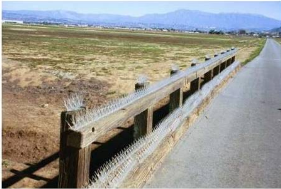
Figure 7-1. Photograph of Bird Spikes on March ARB
