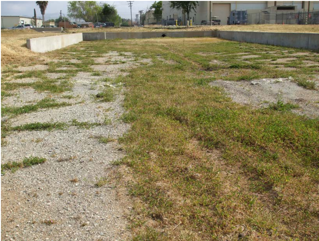
Photo 6 (April 2009): Open concrete basin (Pond #17) at the beginning of the main drainage channel through Survey Area 13. Sediment collected over the gravel base and wetland plants (dominated by Bermuda grass) are growing in the sediment. This is man-made feature and did not meet the criteria for determination of wetlands
